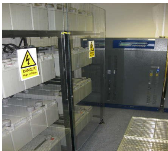
Figure 6 Data Centre power supply backup
